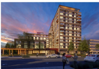
Cairn Pacific's planned Block 294E development at the Con-way site in Northwest Portland will include three mixed-use buildings. (GBD Architects, courtesy of Cairn Pacific)
