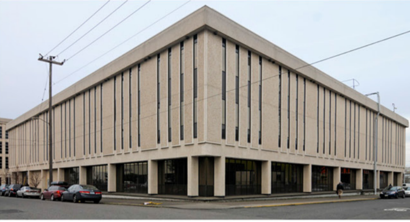
Redevelopment of the Leland James Center in Northwest Portland will be the third project of the second phase of the Con-way Master Plan. (Sam
