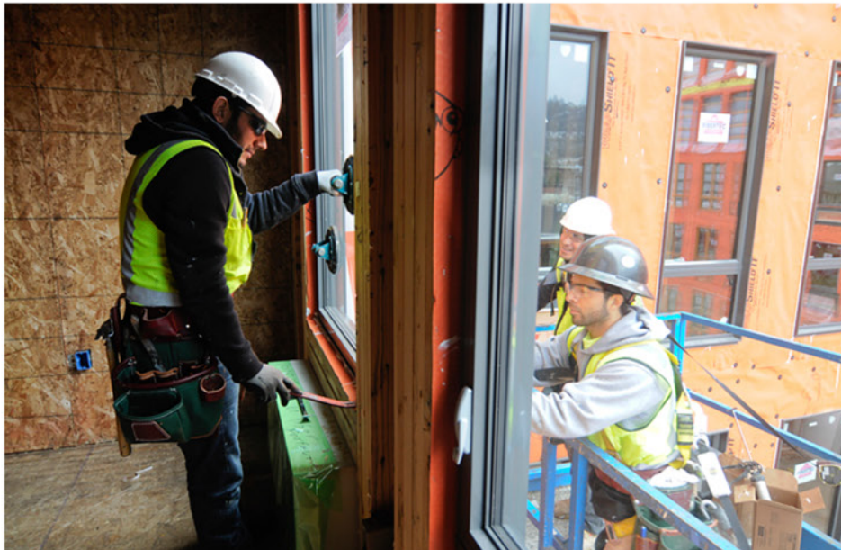
Martin Castaneda, left, and fellow Primo Construction employees install windows on the building's third floor.
