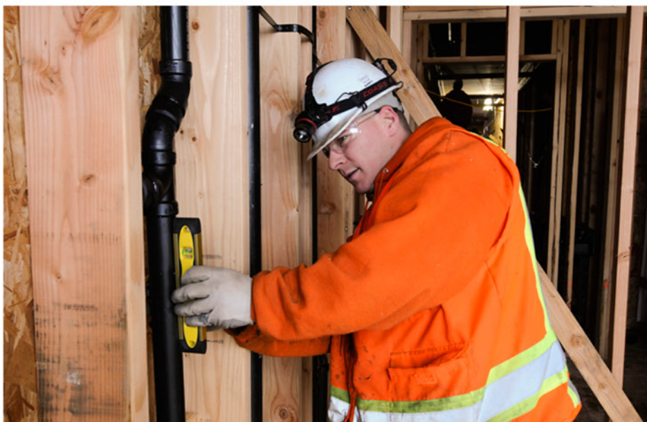
Dennis Anderson, a plumber with American Heating, Inc., checks the alignment of vent pipes.
